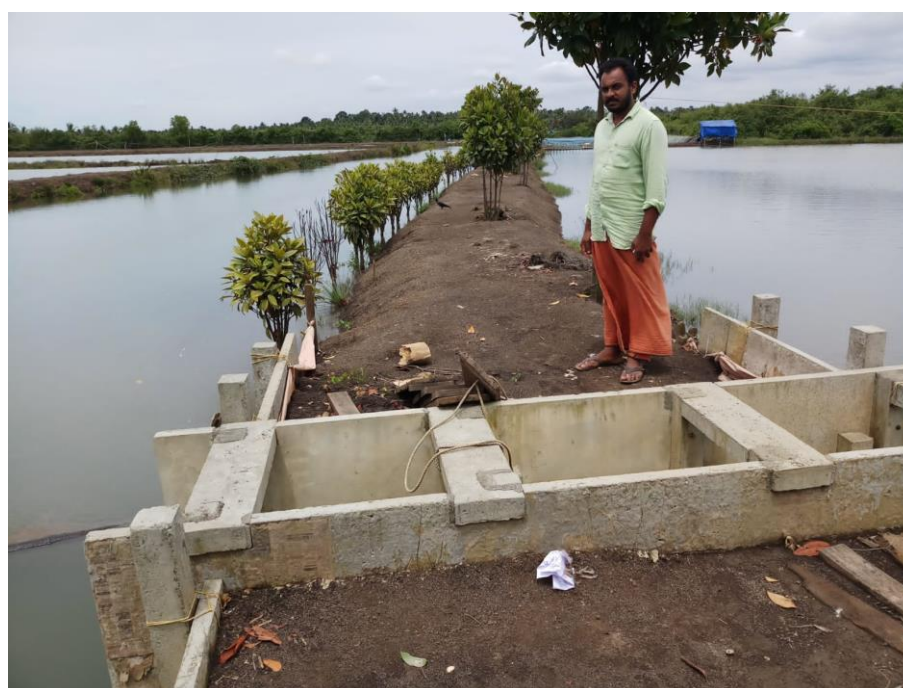
Figure-10 . Inner view of Concrete Sluice built under NAFCC project
