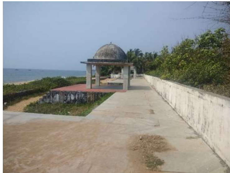
Figure 4.82. Trikannad Walkway and Rain Shelters
