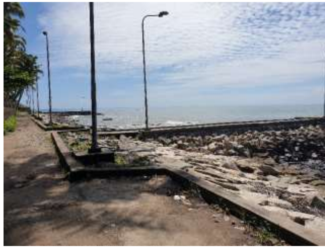
Figure 4.13. Thirumullavaram Beach and Groynes
