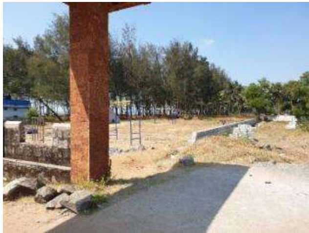
Mannalamkunnu Park Construction
