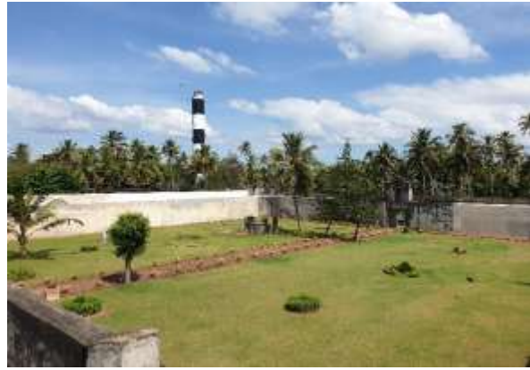
View of Anchuthengu Light house
