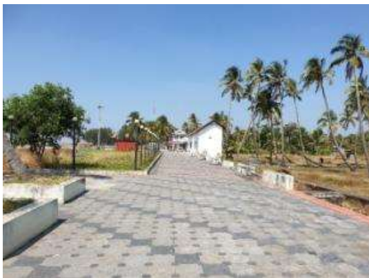
Chavakkad Beach Walkway and Rain Shelters
